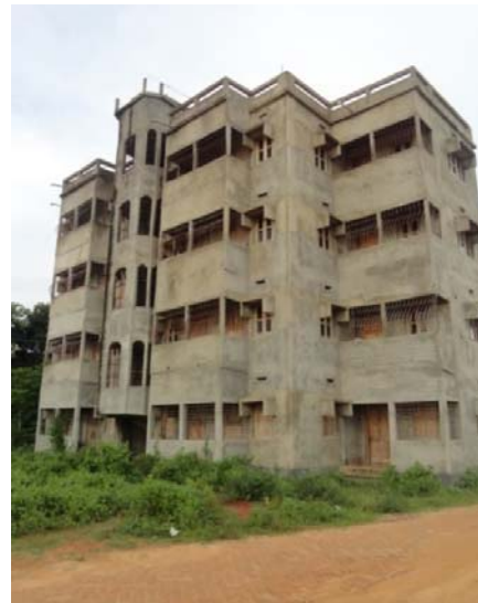
Type-III four storied building constructed at AD Nagar, Agartala
