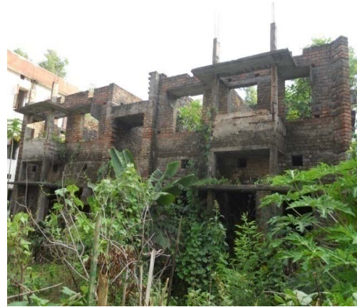
Construction of 9 Type-I quarters in TSR 2 nd Bns remained suspended since long.
