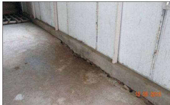
Photograph No. 12 taken on 15-05-2013 Seepage in the floor at PCS
