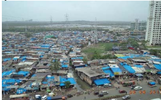
Encroached Shastri Nagar Nalla, Goregaon (W)
