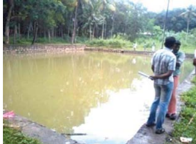
Renovation of ponds
