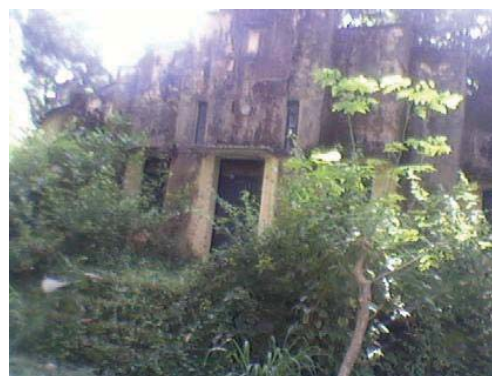
SISI building in dilapidated condition
