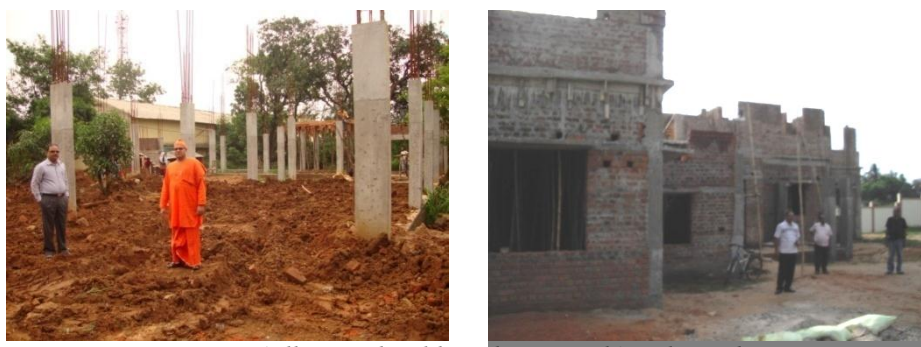
Partially completed hostels at Ranchi and Dumka
