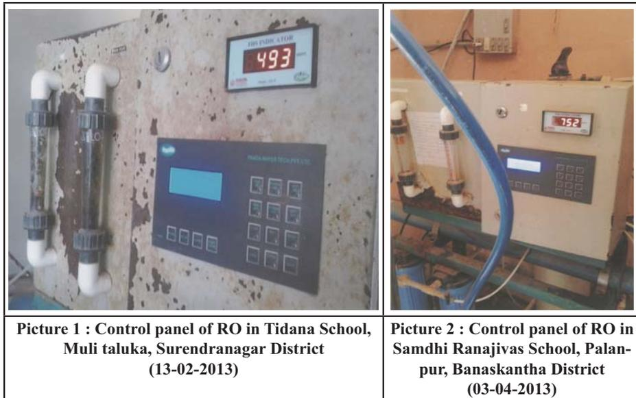
This showed that either the RO System or the display meter was not functioning properly. Thus, the quality of water treated in these systems could not be ensured.
