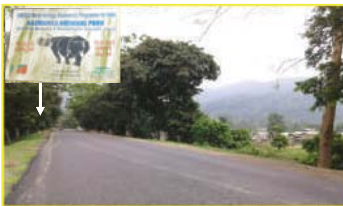
The signage of animal corridor on left side of NH 37 and the settlement of Deosur Chang on the right
