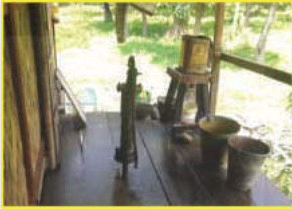
Hand pumps are installed in the camps - strategically elevated so that guards don't have to come down
