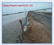
or scouring of road work at any time, if the revetment was not provided. Audit however, noticed (May 2013) during physical verification of road along with the departmental officials that many risk prone stretches were left without construction of necessary revetment works, causing erosion of slopes as can be seen from photograph given above. In reply, Government stated (March 2014) that it had initiated proposal for taking up protection works to road slopes from other grants.
