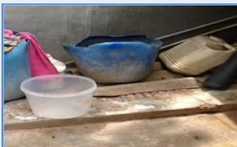
Gram Panchayat: Banda Raviryala Mandal: Hayath Nagar District: Rangareddy Toilet used as store room
