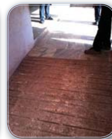
Picture 8 Design of Ramp in Limkhe- da PS, Dahod (03.04.2013)
