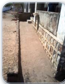
Picture 7 Ramp in Kamboi PS, Dahod (02.04.2013)
