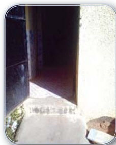
Picture 5 Toilet for CWSN at Chavaj PS, Bharuch (29.05.2013)
