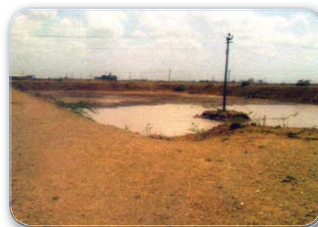
Picture 20 Incomplete SLF developed by GUDC under GERRP at Wankaner, Rajkot District (21.06.2013)
