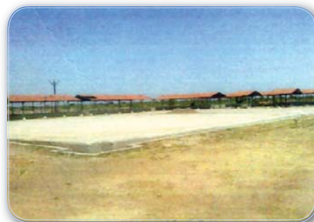
Picture 13 VCP at Thangadh, Surendranagar District (24.05.2013)
