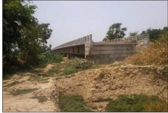
Bridge without approach road on river Khari in Burdwan District
