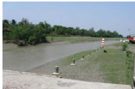
Fig 2:-Lower and upper jetty of FLC
