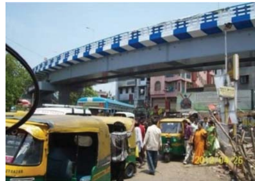
Entry ramp of Dum Dum Road not yet constructed
