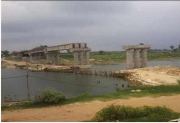
Bridge without approach road on river Mundeswari in Hooghly District
