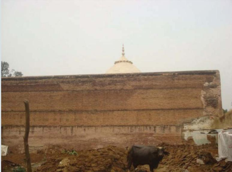
We also noticed cracks in the outer walls, broken stones fixed in the wall, missing designs, use of cement in the wall, seepage, fixing of plastic pipes, and broken jalis.
