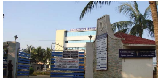
Encroachment of Govt. land by Satabdi Hospital at Tarol
