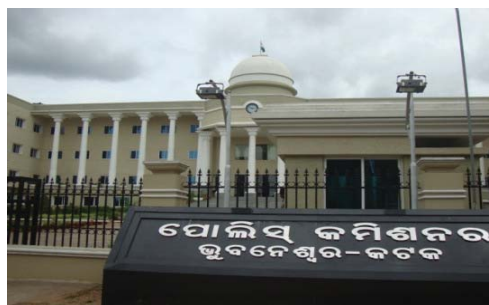
Police Commissionerate office at Bhubaneswar constructed without approval of building plan
