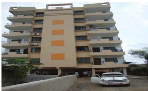
One S+6 building constructed at Ghatikia against the approved plan of S + 4 building
