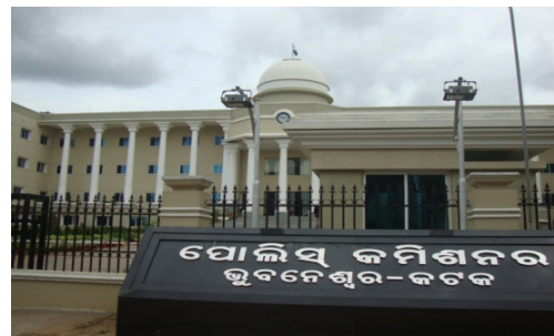
Police Commissionerate office at Bhubaneswar constructed without approval of building plan
