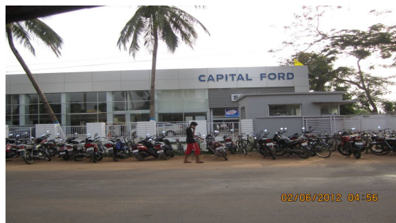
Plot allotted to Blackberry Infrastructure being used as Ford Show room
