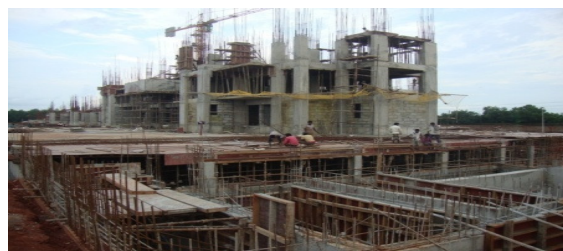
Construction of Vipul Greens at Raisingpur without clearance from MoEF
