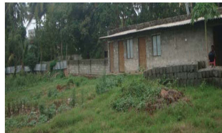
Photograph showing unused land allotted to 'Hotel South Pac Pvt. Ltd'
