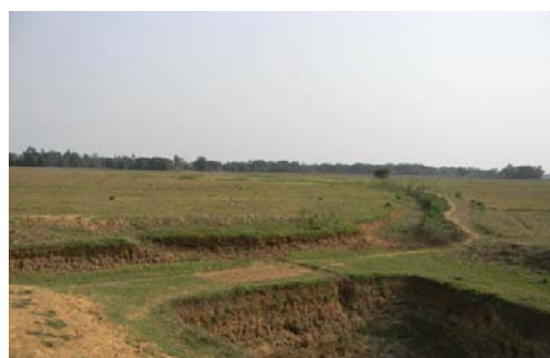
Renovation of Ketuapal Creek
