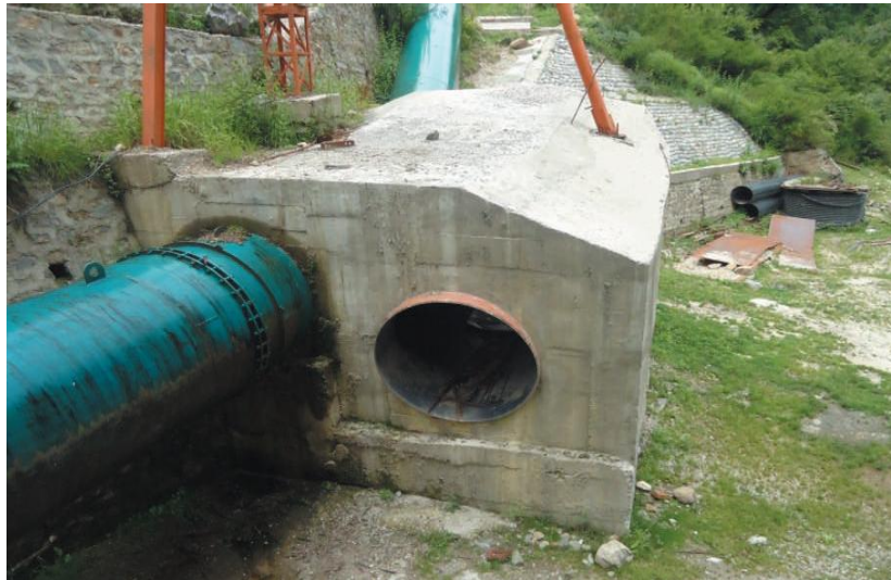
(Penstock of 5MW Toss Hydro Electric Project with scope for 20 MW)
