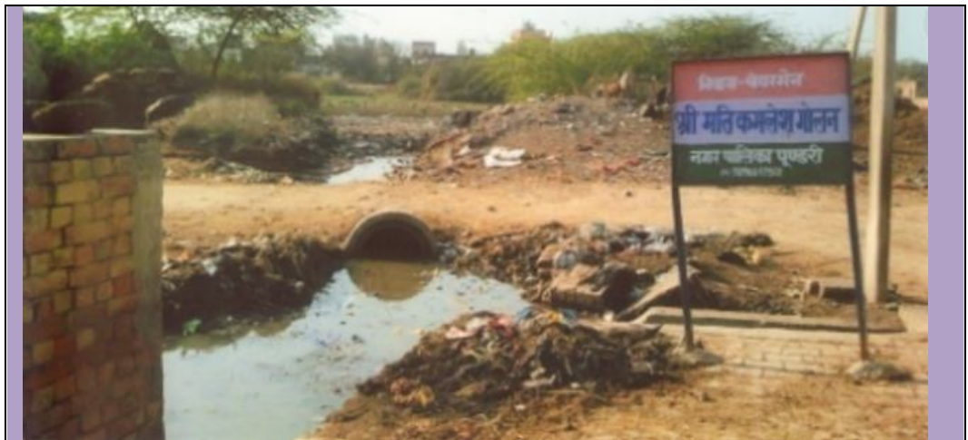
Waste water discharged in katcha drain flowing in the open area in Pundri (10 April 2012)
