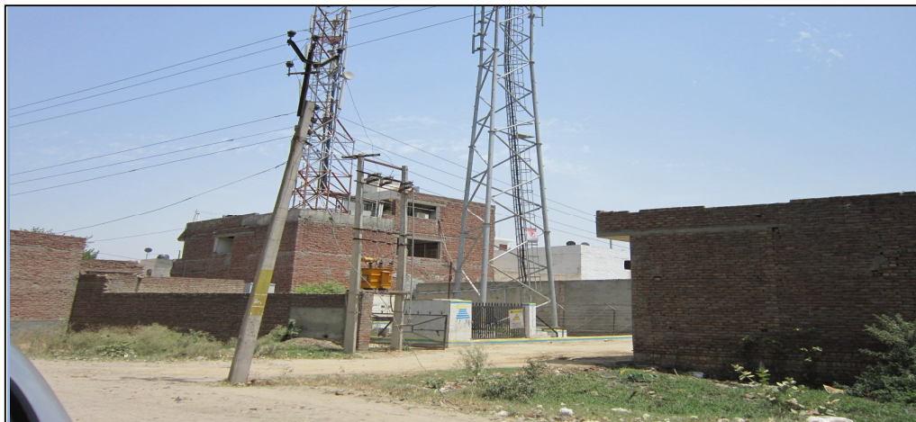
Photo of Arjun Nagar, Panipat, showing the electricity connection in unauthorised colony (13 June 2012)
