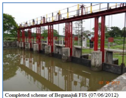
Completed scheme of Begunajuli FIS (07/06/2012)
