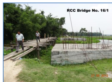
Incomplete RCC Bridge No. 16/1 (27-05-2012)
