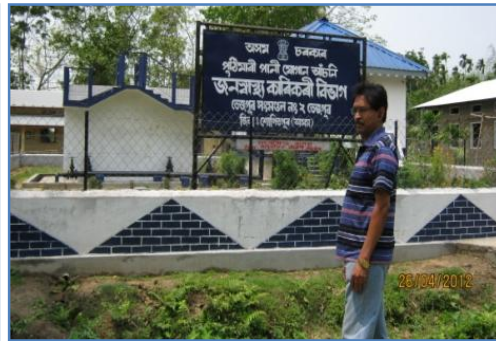
Completed scheme of Puthimari PWSS (26-04-2012)
