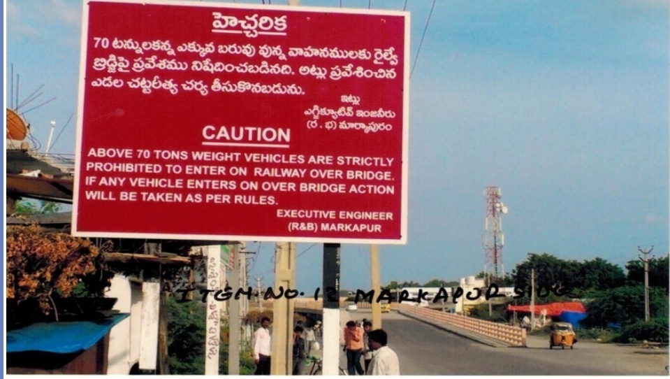
Photograph at ROB at Rayavaram showing warning board to road users for limiting weight of vehicles to 70 tonnes
