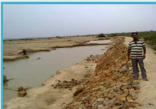
Work ID: 131812802002012770 GP/Mandal/District: Pothugal/Krishnagiri/Kurnool Expenditure incurred: ₹8,71,582 Bunding was completed without any revetment
