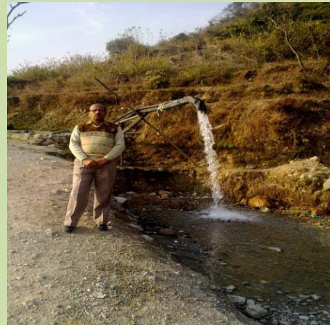
Dewatering activity in progress in T-1
