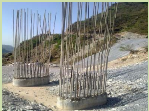
Pier P 19 in dismantled condition
