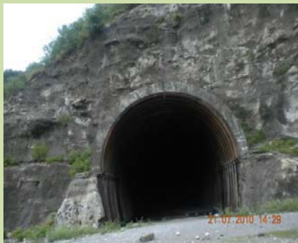
Tunnel T-2 abandoned
