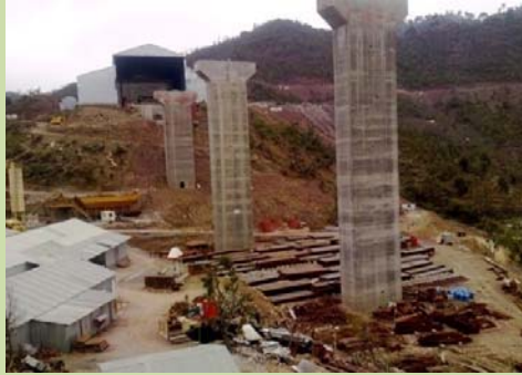
Via duct portion of Chenab Bridge- photograph of suspension period
