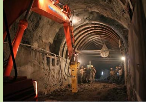
TUNNEL T1/P1 REZIFICATION WORKS IN PROGRESS (PHOTO ON 21/07/2010)
