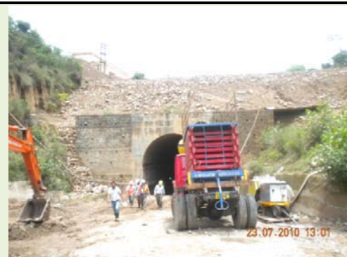
Reconstruction work of T1 portal 2 in progress
