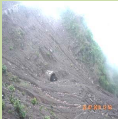
Portal T-7 P2, which was abandoned
