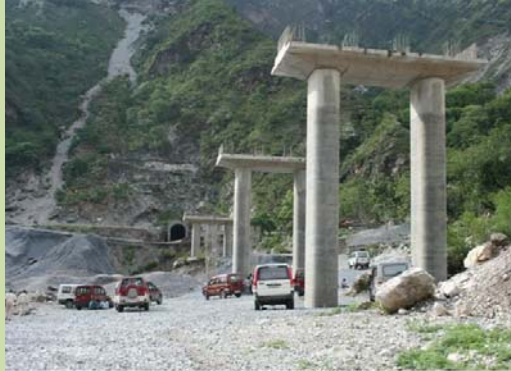
View of Anji Bridge site (22.07.2010)
