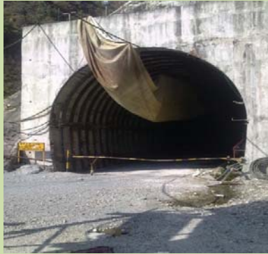
Tunnel T-5 during suspension period
