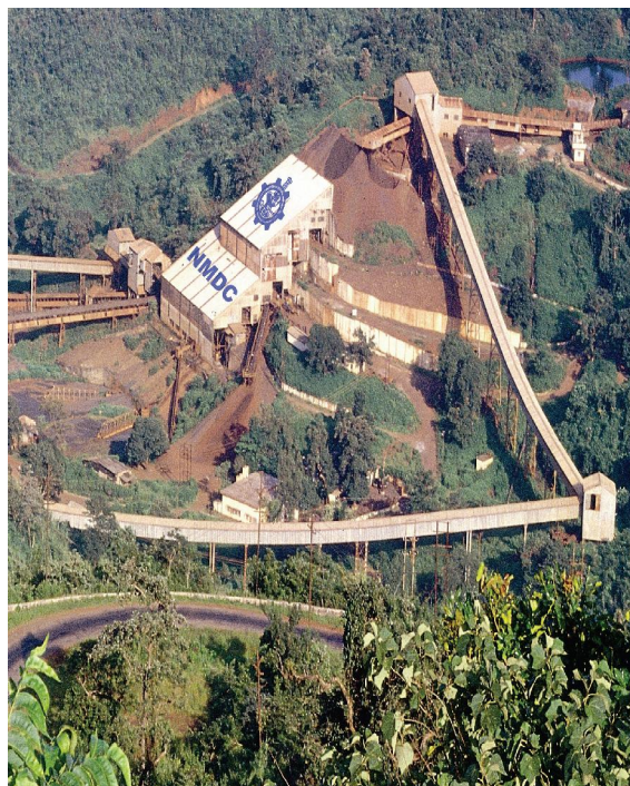
Fig 2: Aerial view of downhill conveyor at Bacheli
