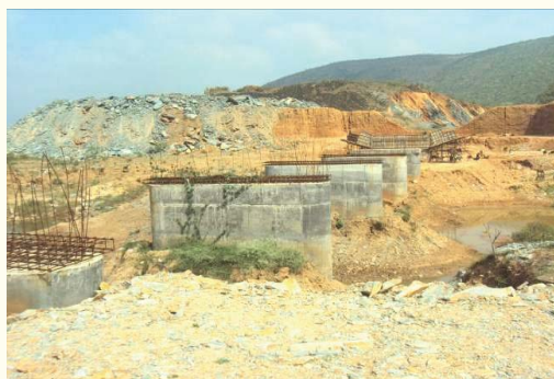
Non completion of CM & CD 21 works (Aqueduct)
