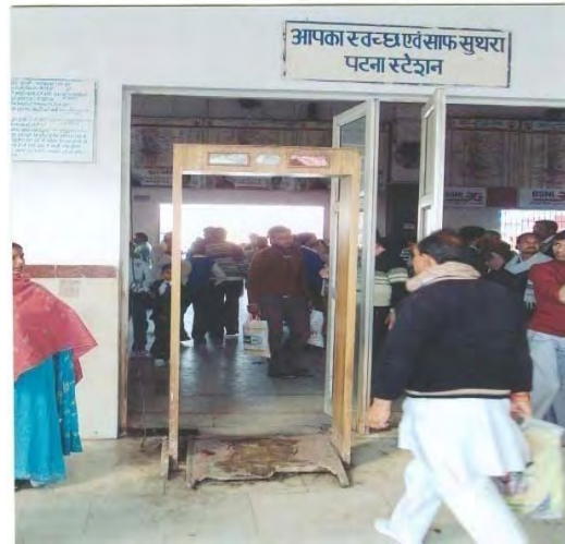
Gap near DFMD at Patna station in ECR
