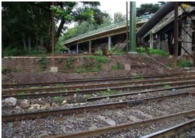
Ghorouri Yard. Pune open from all sides
