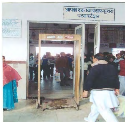
Gap near DFMD at Patna station in ECR
