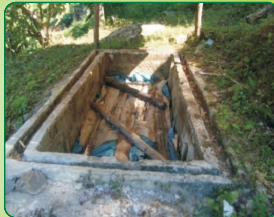
Defunct vermin compost pit under Poklok Denchung GPU
