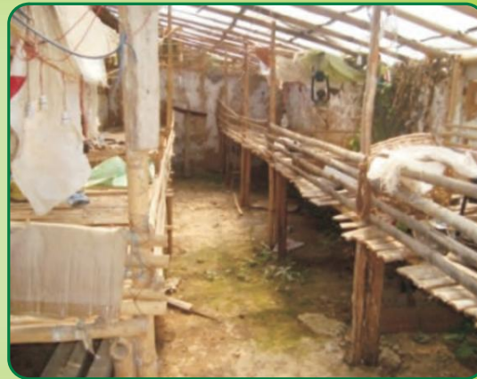
Empty poultry shed at Poklok-Denchung GPU
