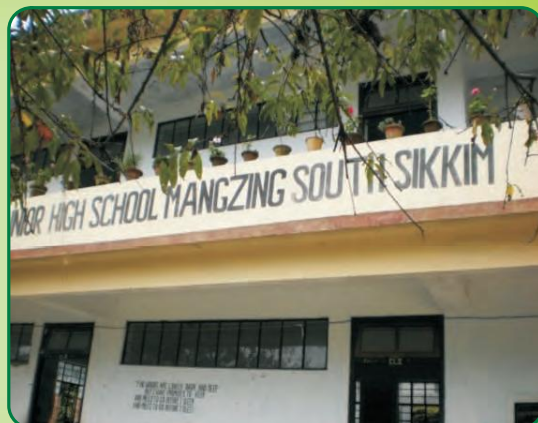
A good school building of Mangzing JHS under Niya Mangzing GPU
