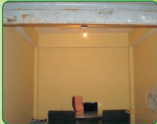
Shops are being utilised as Office by the UDHD
