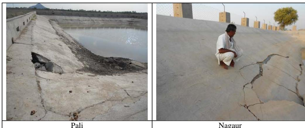
Photographs showing defective water sources with leakage/cracks (Pali and Nagaur)
