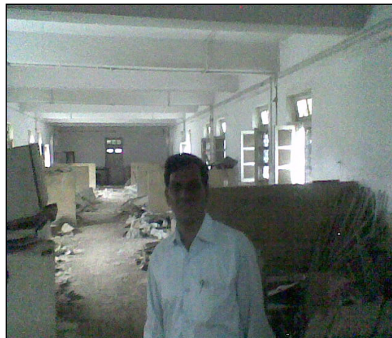
Twenty one bedded ward used for storage of waste material
