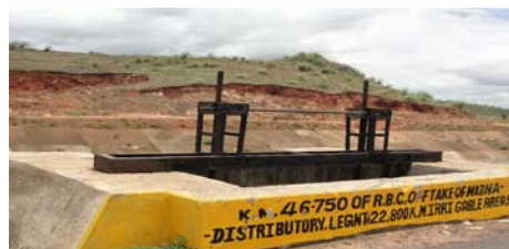
View of availability of CNS material at RD 46.750 km of RBMC
