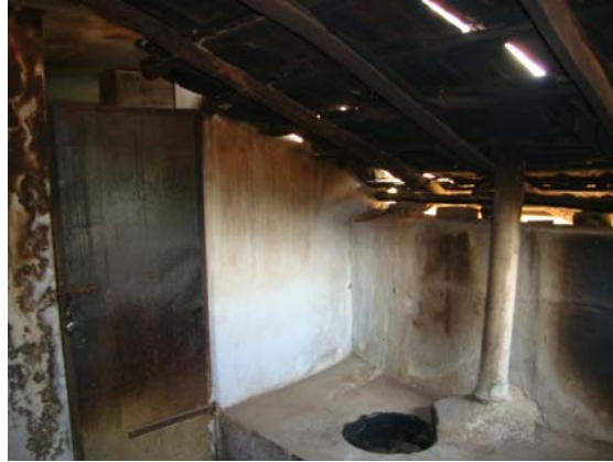
ALPS, Kinavallur- Kitchen adjacent to Toilet
