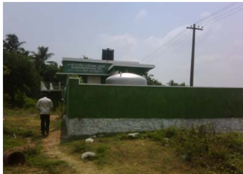
ARWSS Parali – Idling water treatment plant
