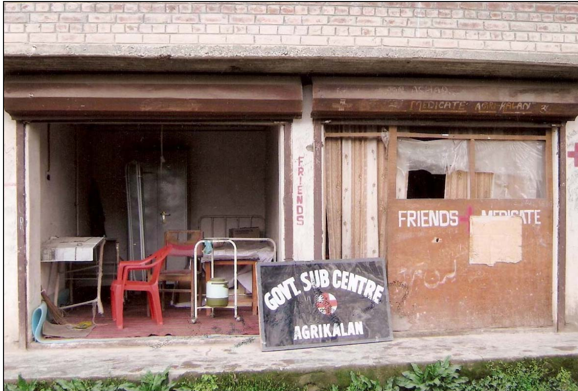
Sub-centre Agrikalan (Pattan) housed in shops
