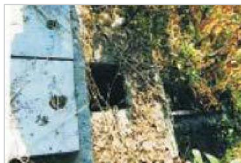
Overflowing of sewage from Septic Tanks without soak pits in Bilaspur town (6 December 2011)
