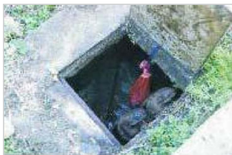
Overflowing of sewage from Septic Tanks without soak pits in Bilaspur town (6 December 2011)
