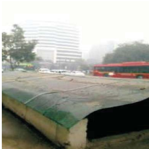
Covered subway entrance after re-filling
