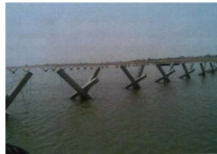
RCC Jack-Jetty System (Taken from PCN)
