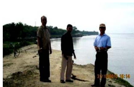
Eroded newly constructed embankment
