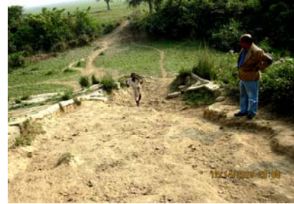
Incomplete ramp of Rangmahal garh (14 December 2010)
