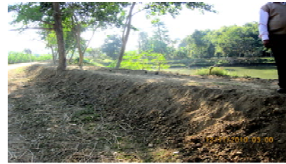
On going dowl bund of Bagjap Ph II (17 December 2010)
