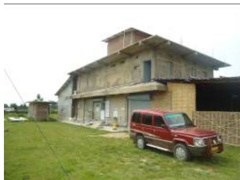
Unauthorized erection of mineral water plant in a portion of the land
