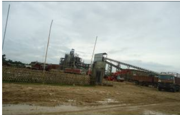
Agricultural land alienated to CALCOM Cement Ltd.
