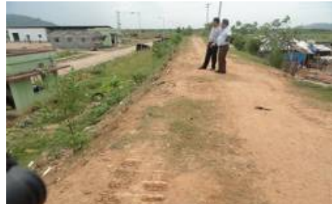
EARTHEN BUNDH AROUND THE COMPOST PLANT (July 2011)
