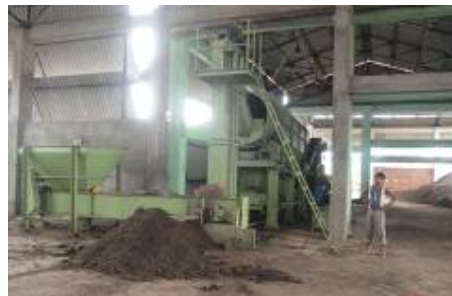
COMPOST PLANT (July 2011)
