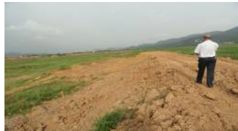
EARTHEN BUNDH AROUND SLF AREA (July 2011)
