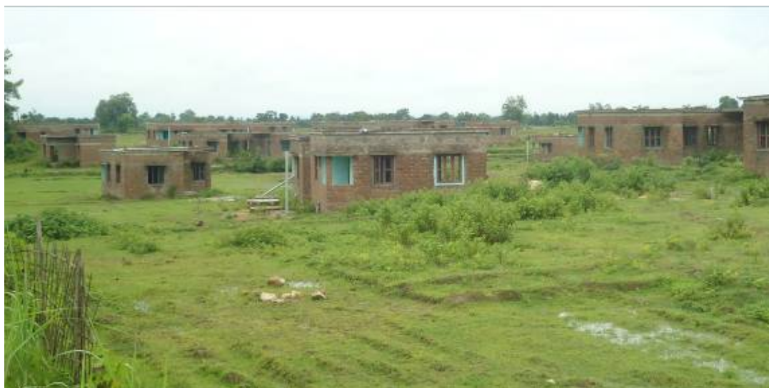
Incomplete houses for PAF (July 2011)
