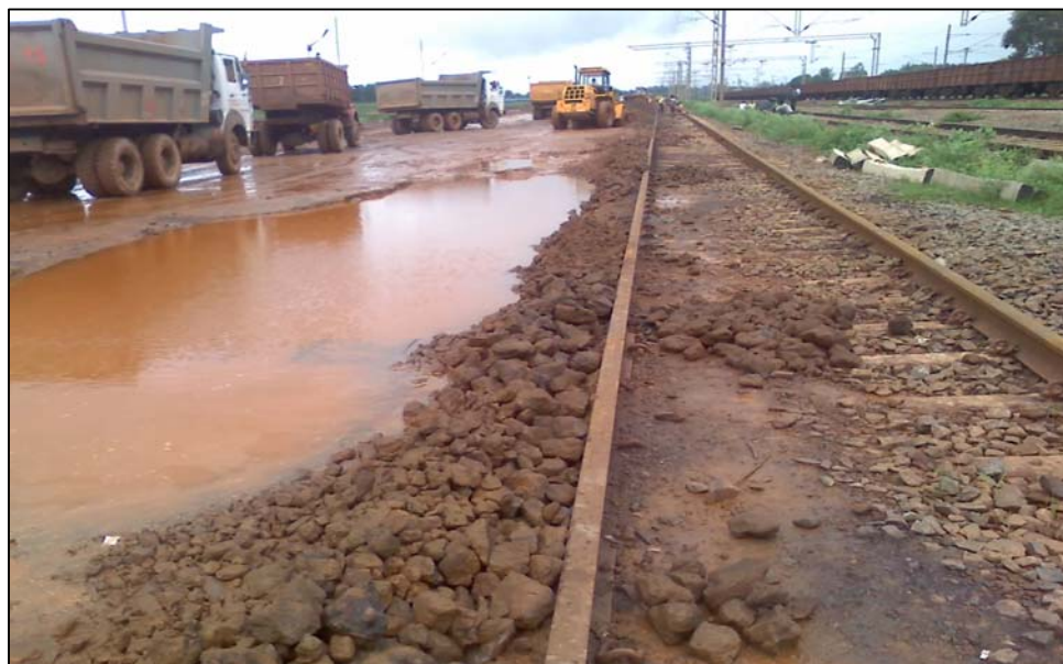
Broken concrete basement at Jagdalpur goods shed
