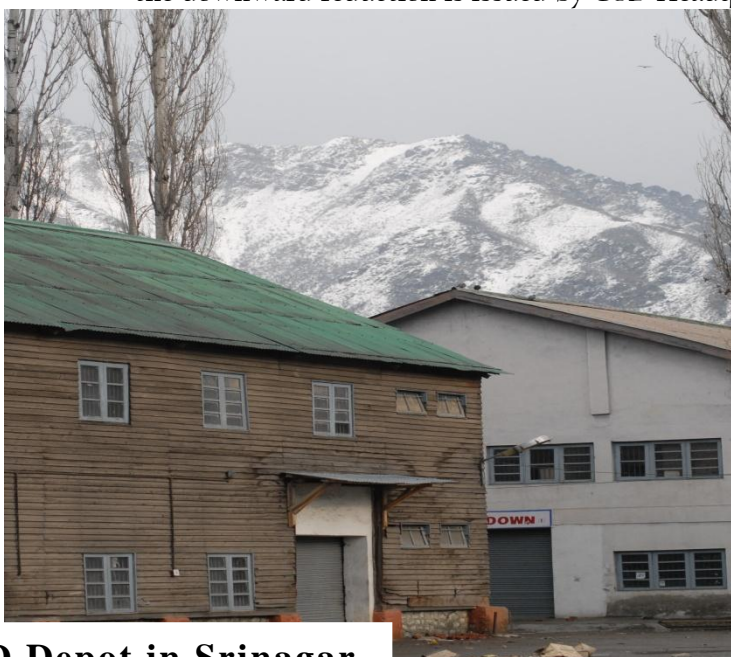
CSD Depot in Srinagar
