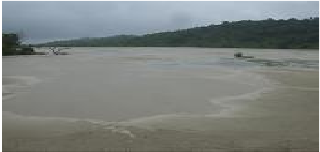
Tailing Dam (September 2010)
