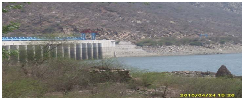
Water level of Bisalpur Dam stands at 302.820 metre (24.4.2010).
