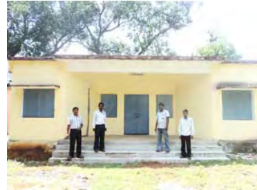
Idle DDL building at paralakhemundi
