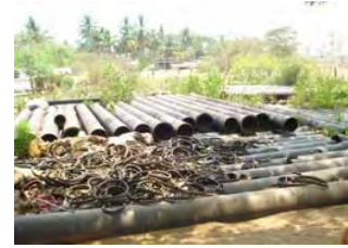
CI pipes and joints lying idle since March 2008
