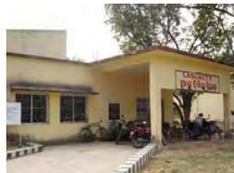
Casualty Building at Sundargarh Hospital lying idle since September 2008
