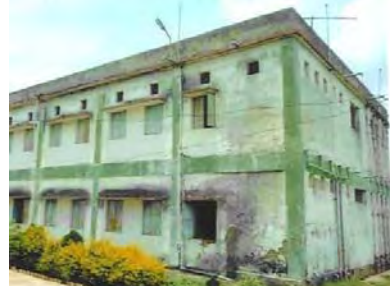
Hostel Building constructed for Government Women's college, Sundargarh lying idle
