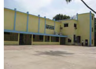
Inadmissible project: Town Hall, Berhampur on which ₹ 15.50 lakh spent under BRGF
