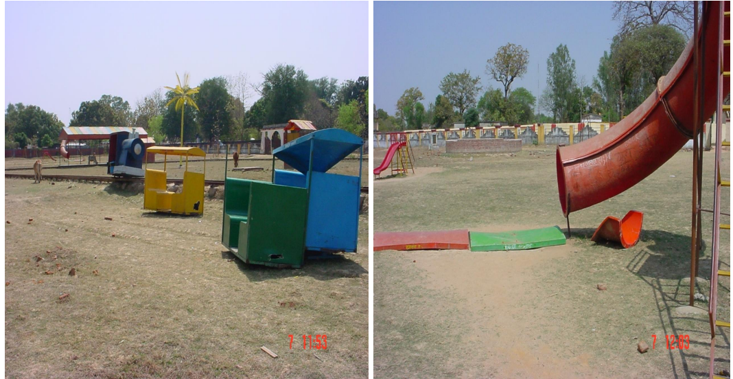
(Photos showing incomplete/damaged work of construction/beautification of Park at Simdega)
