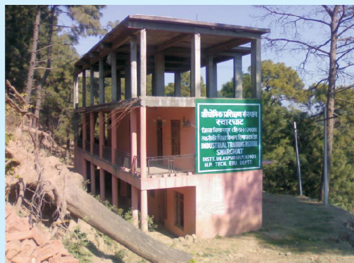
Partially completed GHB at Swarghat, Bilaspur District
