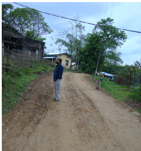
Road from PWD Arunachal to Akrum Ali's House near river Barak under NREGS 2008-09 in Tupkhana GP under Silchar Dev. Block/11 March 2010
